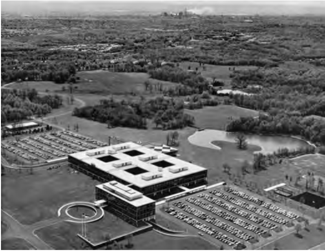
Abb. 62 Skidmore, Owings & Merrill (SOM): Verwaltungsgebäude Connecticut General Life Insurance Company, Bloomfield, Connecticut (1954–57).
